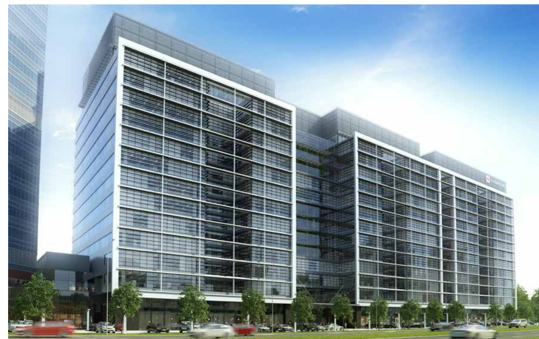
EUROCENTRUM OFFICE COMPLEX
